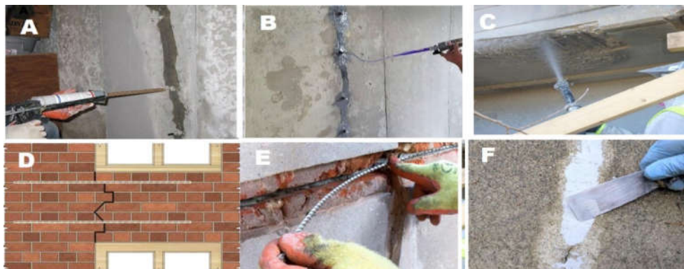
Figure 1 a) Grouting using polymer injections, b) Epoxy Injection using epoxy paste c) Shotcrete method of crack repair d) Crack Stitching using metal plates e) reinforce a cracked wall, and f) cementitious filler or sealant.
