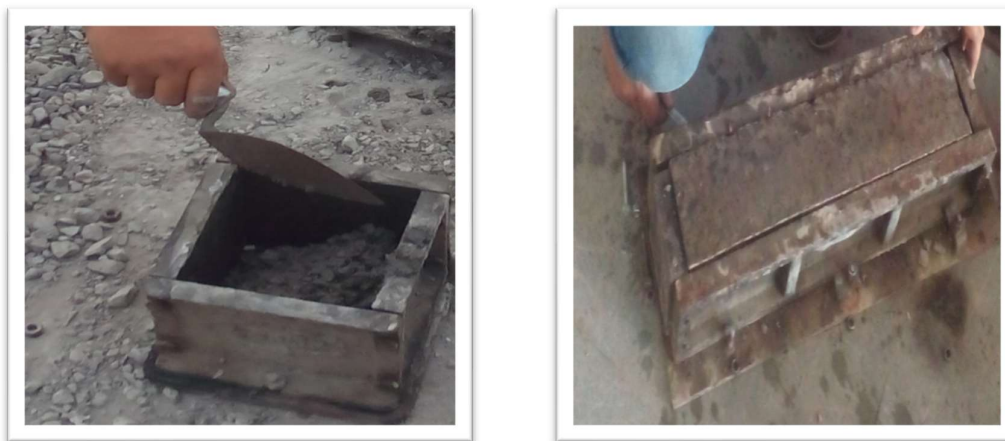
Figure 4.3: Cubes & beam casting.
